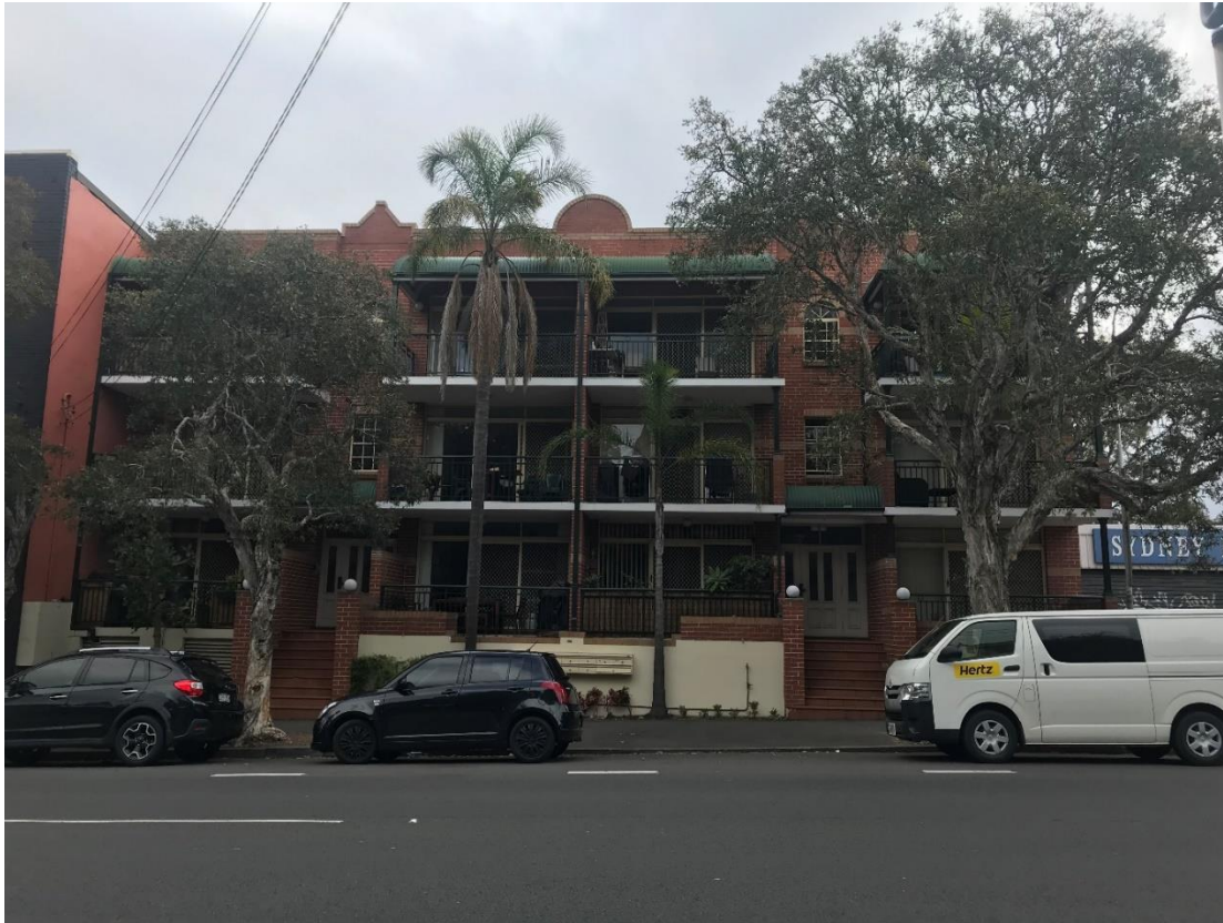
Figure 8: View of adjoining residential flat building at 593-601 Elizabeth Street
