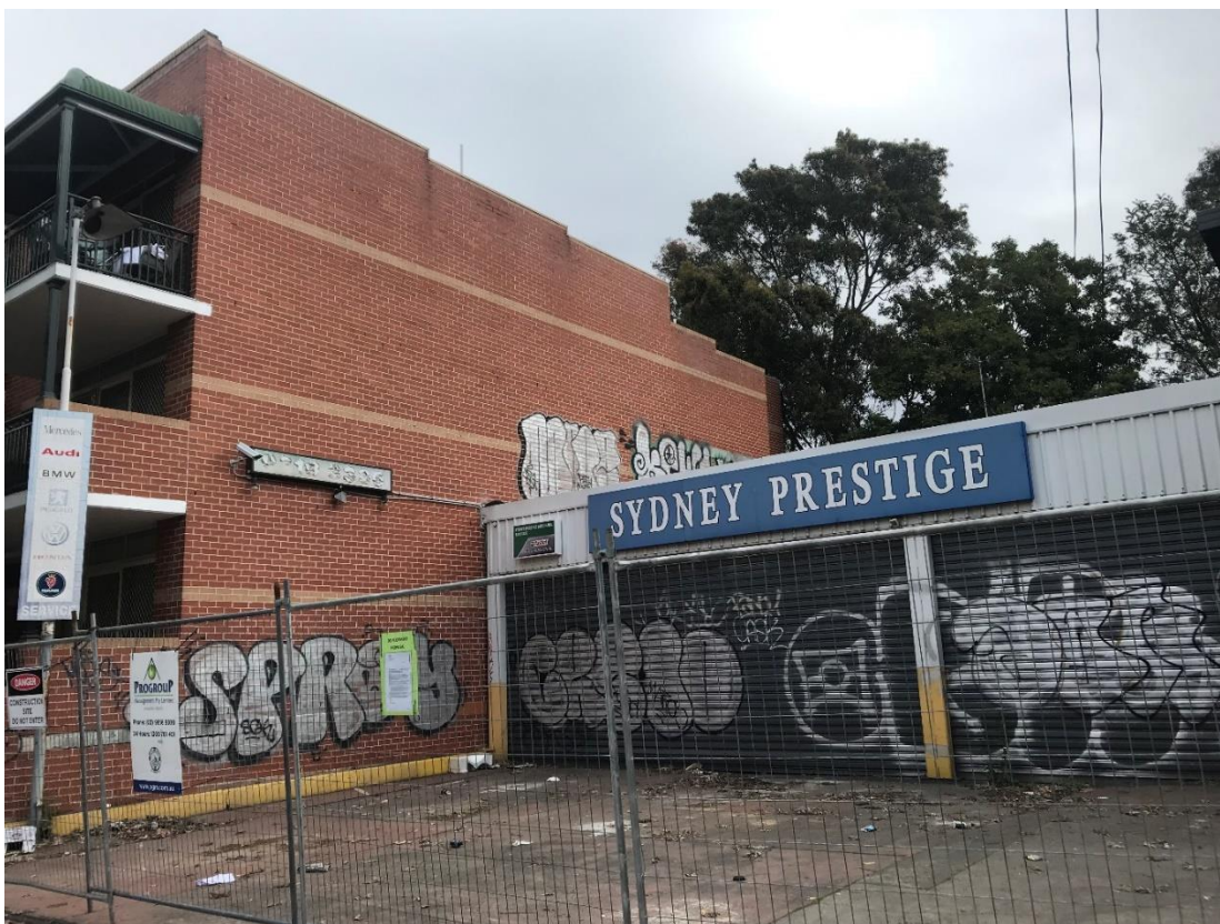
Figure 9: View from Elizabeth St of site and adjoining residential flat building at 593-601 Elizabeth St
