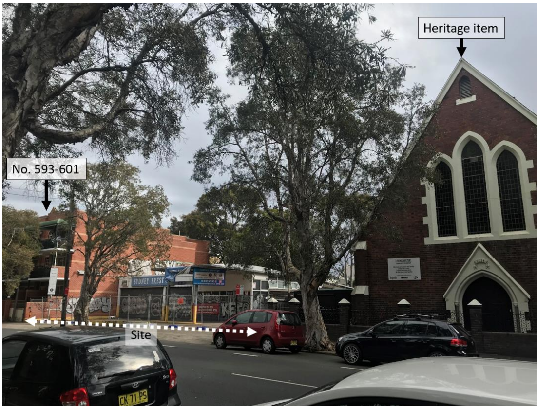
Figure 3: Looking south-west from Elizabeth Street
